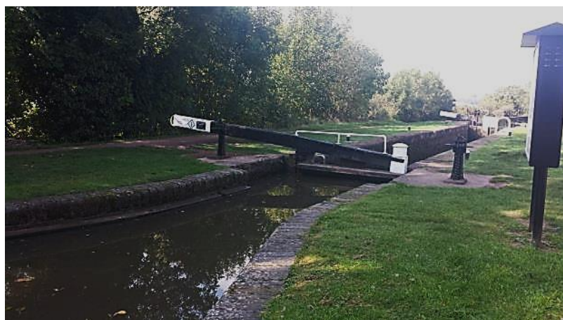
Fig 2 below View of Lock 1 Droitwich Junction Canal
