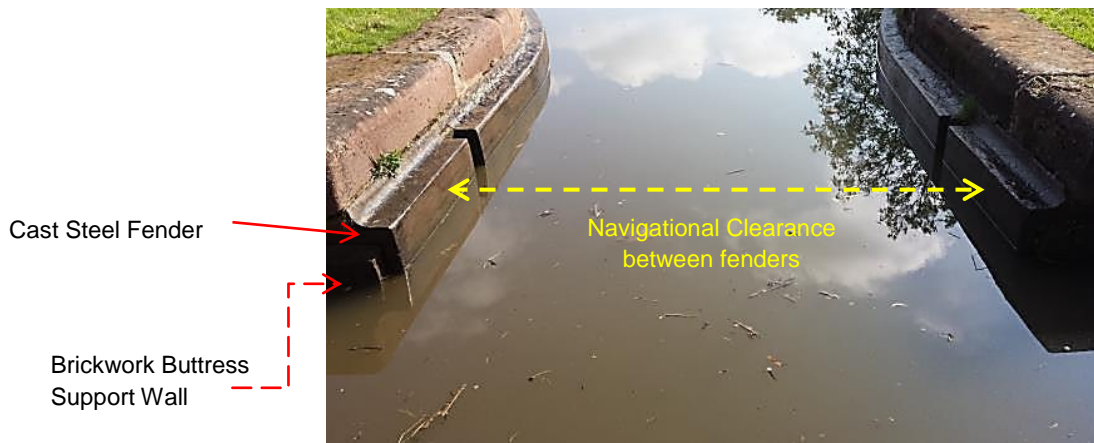
Fig 1 View of steel fender
